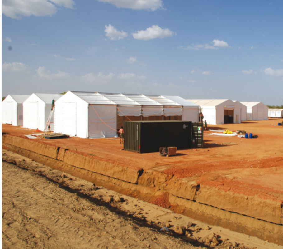
Camp Ciara under construction.
